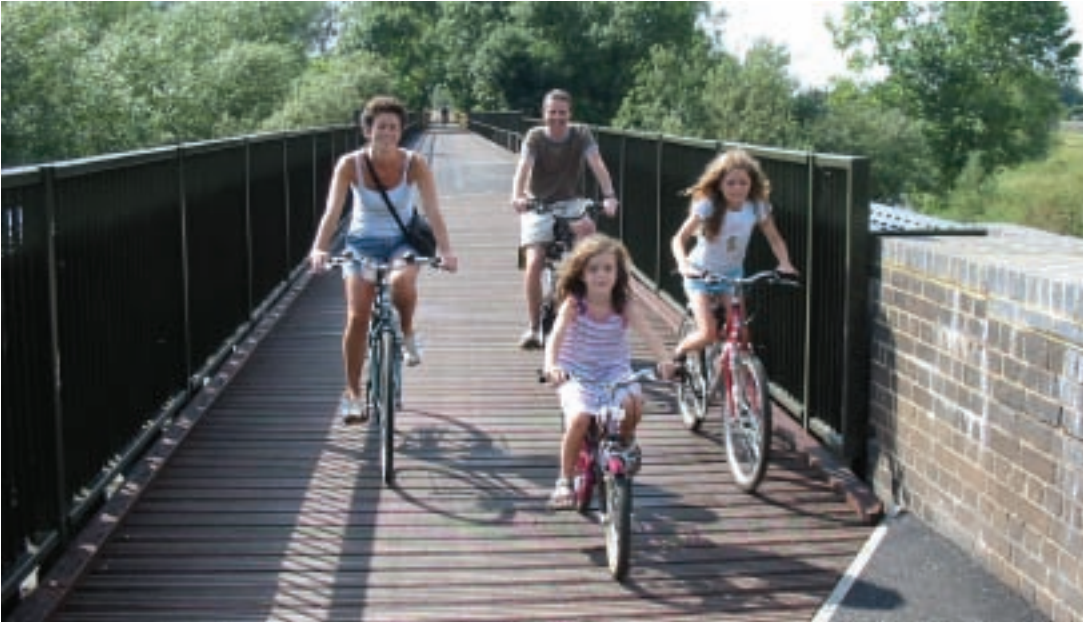
Family using a repaired bridge across the River Ivel at Blunham, Beds., on Route 51 of the National Cycle Network. Photo: Forest of Marston Vale
